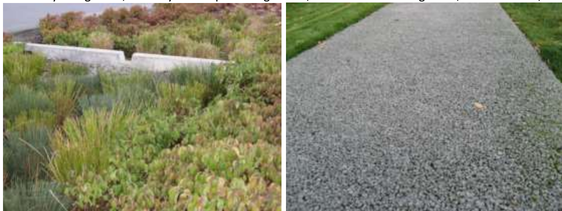
Biodiverse community Raingarden, Portland; and permeable pavement feeding rainwater into a lawn, Seattle.
