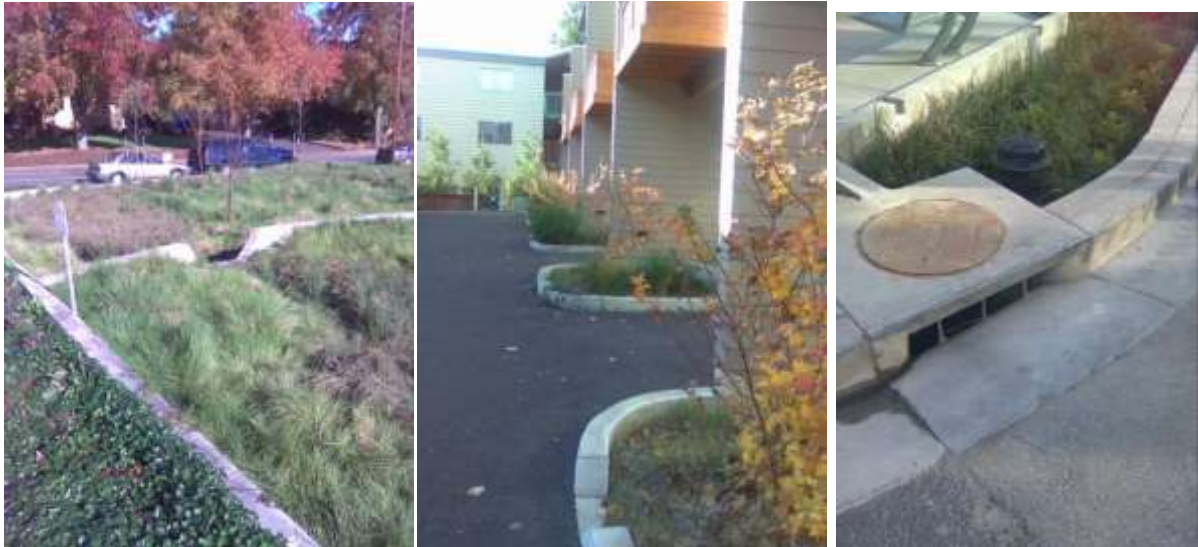
Community Raingarden, an array of unit plot Raingardens, and a kerbside Raingarden, all in Portland, USA.
